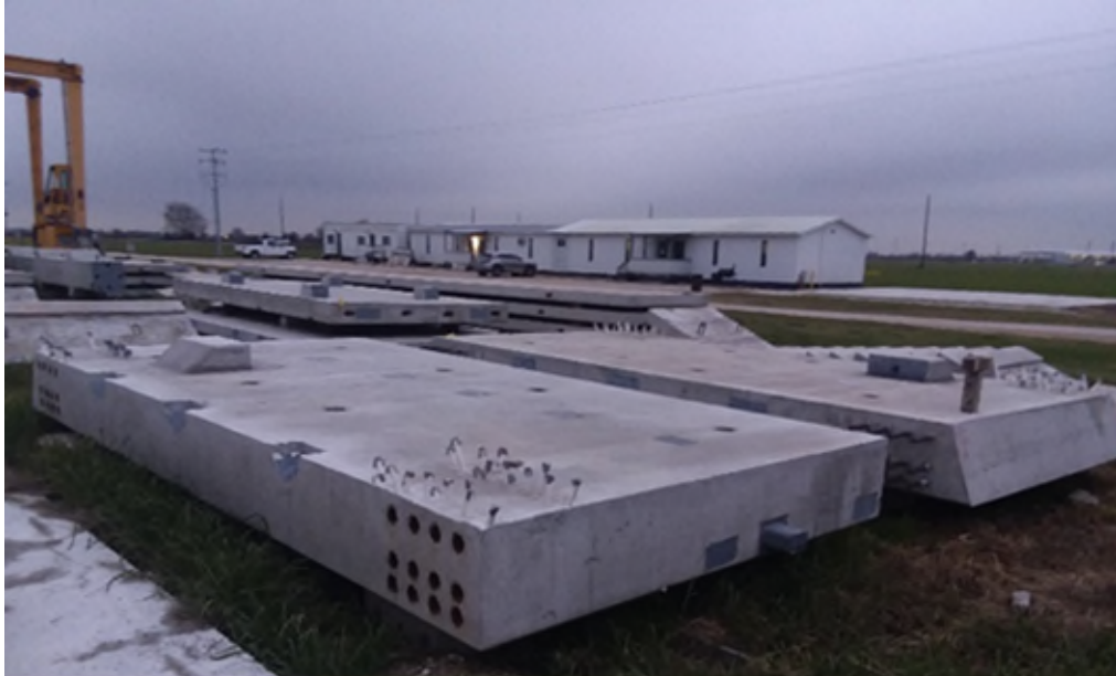
Typical Shear Walls in Storage
