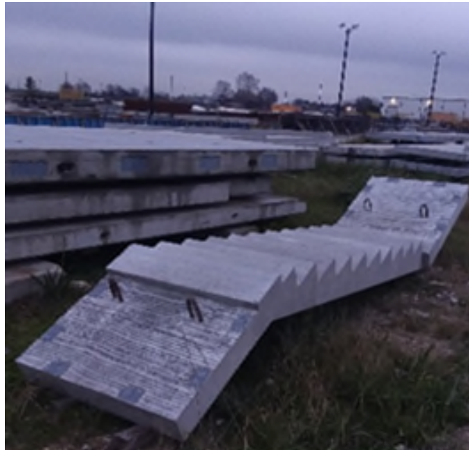
Typical Stairs in Storage
